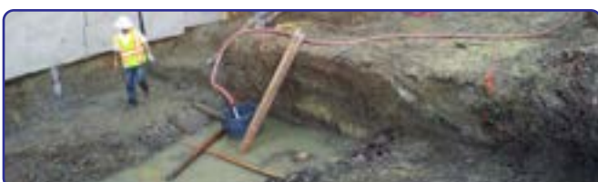
Construction dewatering monitoring
